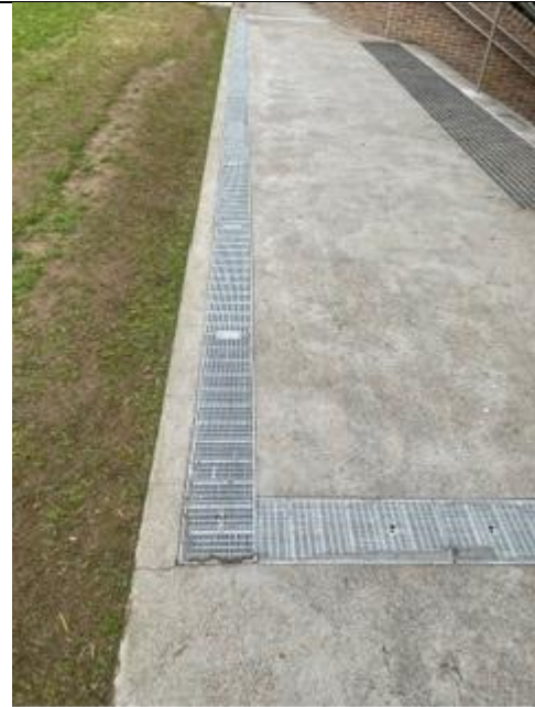
Photo 6: Stormwater collection drains at top of staircase
