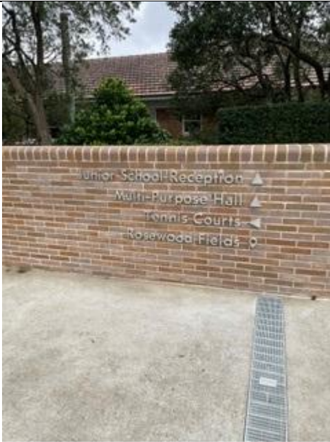
Photo 9: Installed gutter drain at top of staircase
