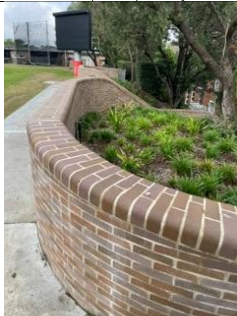
Photo 4: Completed staircase brickwork and landscaping
