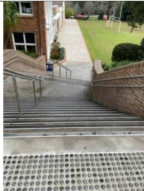
Photo 8: Photo on top of staircase
