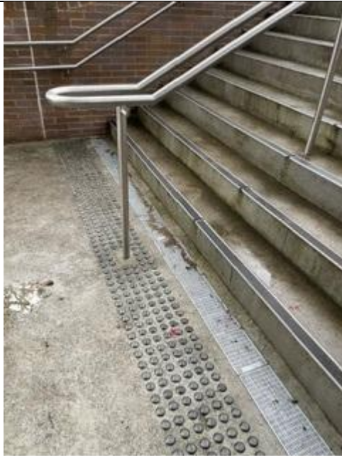
Photo 13: Drain at base of staircase
