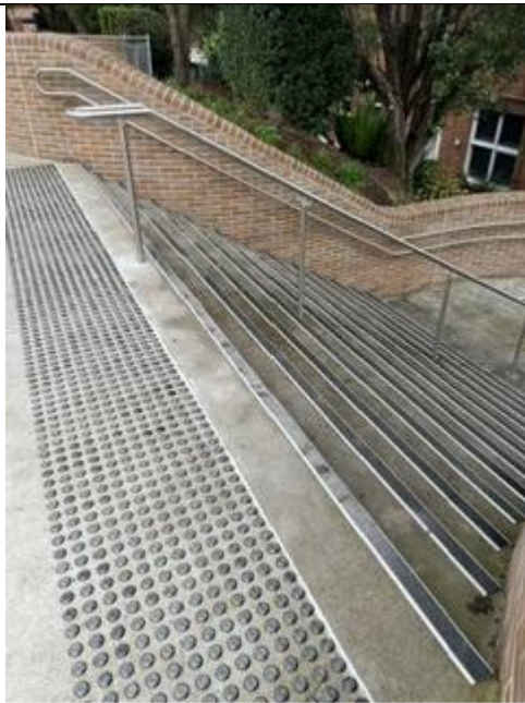
Photo 7: Completed staircase construction works
