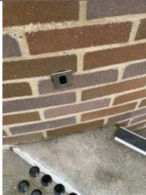
Photo 10: Staircase built in lighting
