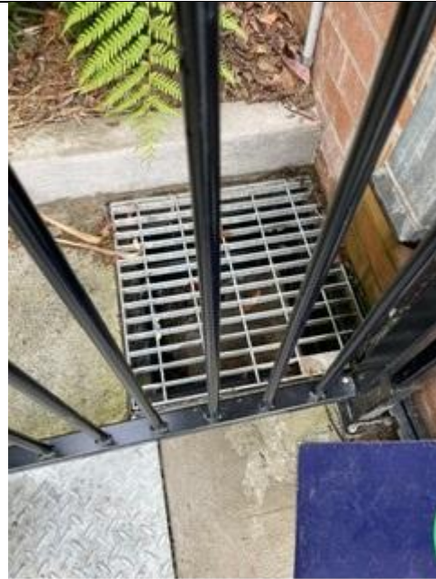
Photo 14: Reticulation of drainage from staircase to main stormwater drain
