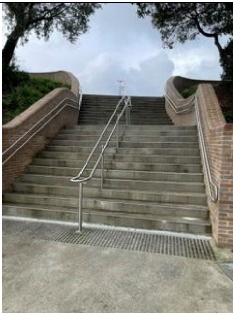
Photo 15: Photo at base of staircase
